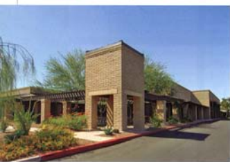
Top: High ceilings and skylights showcase the furniture, accessories, lighting and art at John Brooks, Inc.'s new, spacious showroom.
